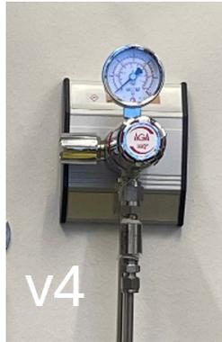
5. Fully remove the load lock bolts and flange when LL pressure reads 1000 mbar – insert sample (gloves must on) – stop the nitrogen flow via v4 – close the Load lock bolts (one up right, one down left) and flange. Hand tighten the two bolts instead of using a wrench, to avoid over-tightening.
